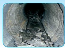
Descaling large diameter pipework - 200 lpm / 1000 bar
